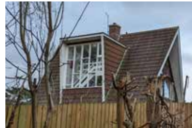
Scandinavian style roof - Gabled high pitched roof with clay tiles & hung tile dormer
