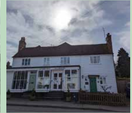
Figure 06: Sandhurst tearoom - a ground floor cafe with residential unit above, with little setback from the main road.
