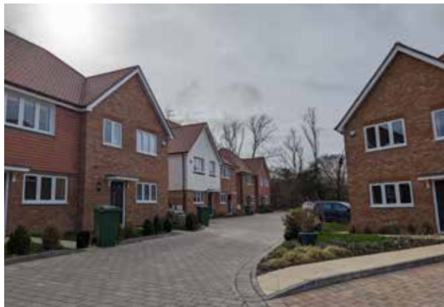
Figure 42: Local example of a cul-de-sac development where buildings, mainly 2-2.5-storeys, are set along a meandering streets with limited boundary treatments, mainly small grass verges and flowerbeds, Old Orchard.
