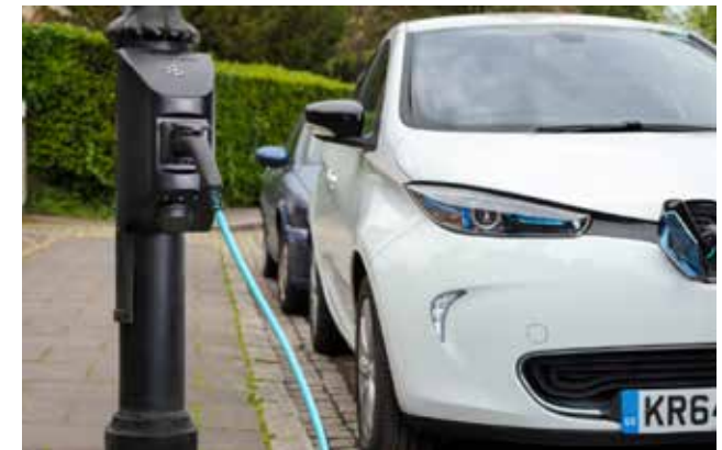
Figure 27: Example of on-street electric vehicle charging points.
