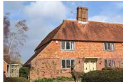
Cat-slide roof with kent peg tiles and brick chimney
