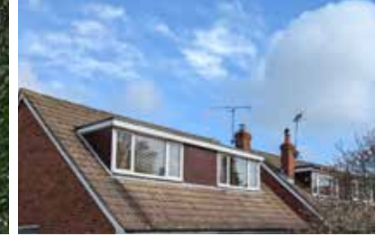
Gabled tiled roofs & hung tile dormer
