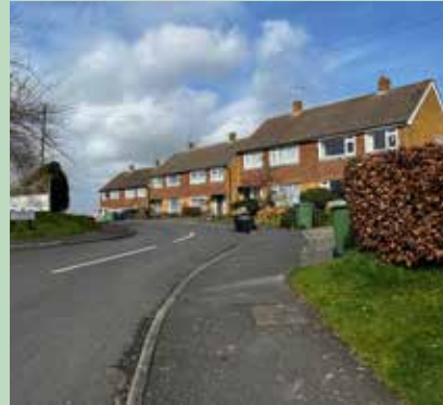
Figure 12: Semi-detached houses built with a mixture of yellow and red brick along Tanyad/Poundfield Road, offering active frontages that frame the intersection.
