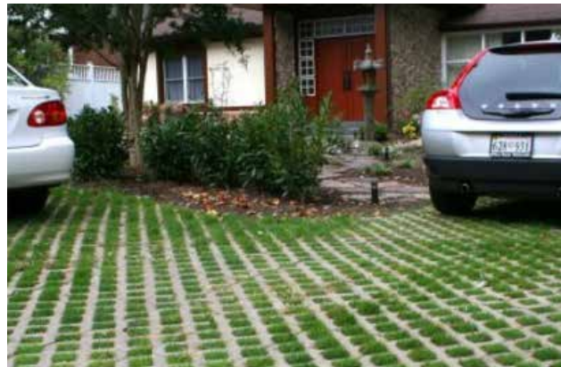
Figure 22: Example of permeable paving in driveways that helps minimise surface water run-off, whilst improving the rural environment and biodiversity of the area.
