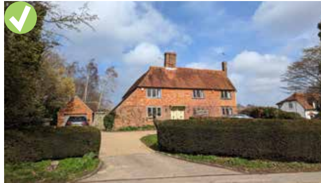
Figure 51: Local example of a south facing property (approx. 30 degrees) that maximises the solar gain, whilst plantation to the north offers protection from cold northerly winds, Queen Street.
