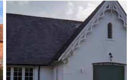
Cross gabled roof with slates & decoration
